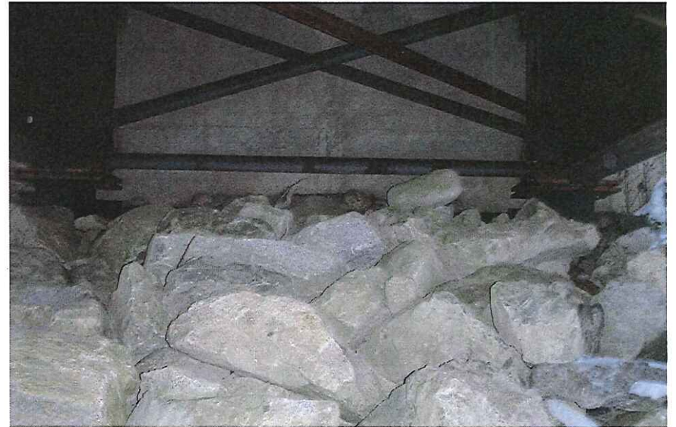
CK-2050 Abutment Left Bank
