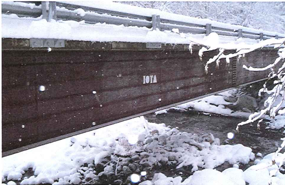
CK-2050 Crossing Upstream
