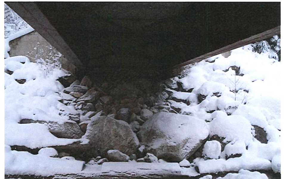
CK-2050 Abutment Rightbank
